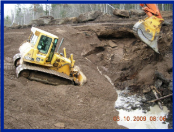
Heavy equipment working on the road.
