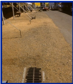
A storm drain at the fairgrounds.
